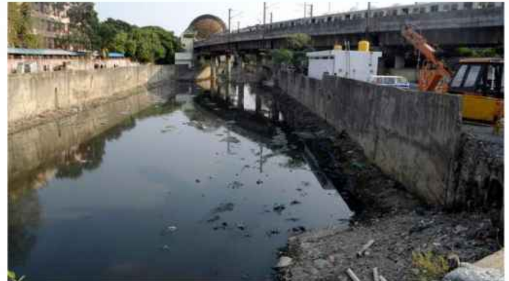
The Water Resources Department will undertake a pilot project to restore the Buckingham Canal on a 2.9-km stretch, between Swami Sivananda Salai and Dr. Radhakrishnan Salai. | Photo Credit: M. VEDHAN
