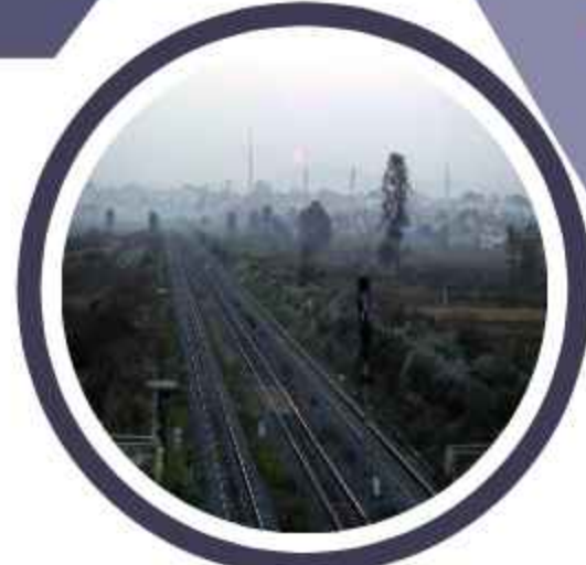
3 rd Line Railway Track From Tambaram Chengalpattu
