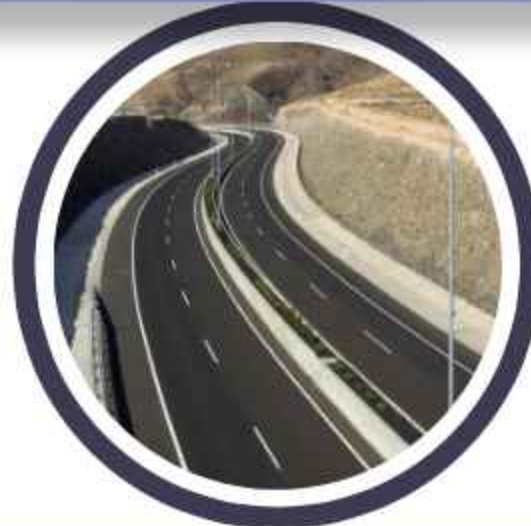
2 Lane to 4 Lane Road (GST to OMR) (Nellikuppam Road Expansion )
